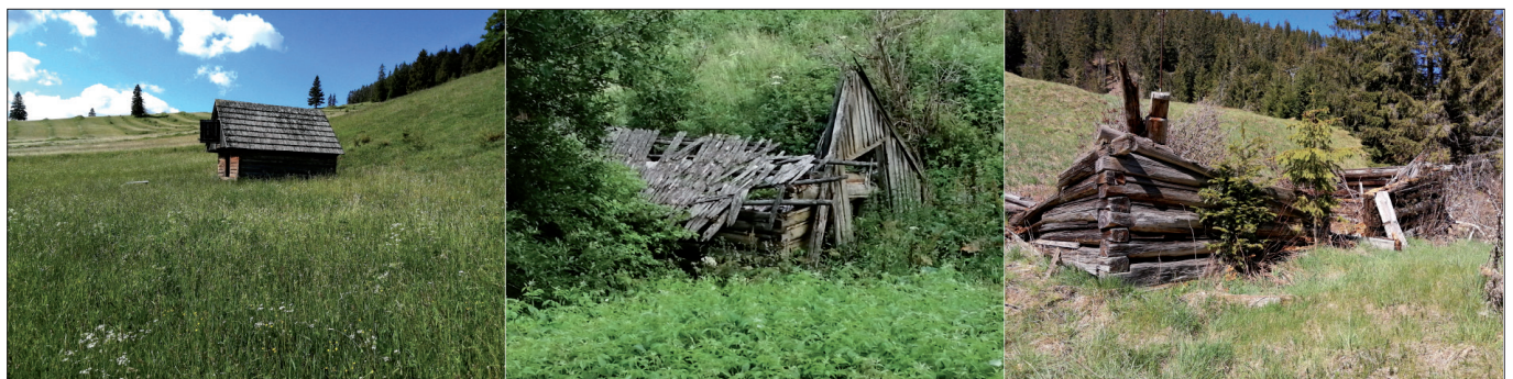
Fig. 6: Example of different stages of decay of haylofts in the Upper Liptov Region – from left to right: (a) Preserved hayloft in a complex of hay meadows with high biodiversity in Liptovská Teplička – type I.; (b) Damaged hayloft in the cadastre of the Nižná Boca – type II.; and (c) Remnants of the hayloft in Nižná Boca – type III
