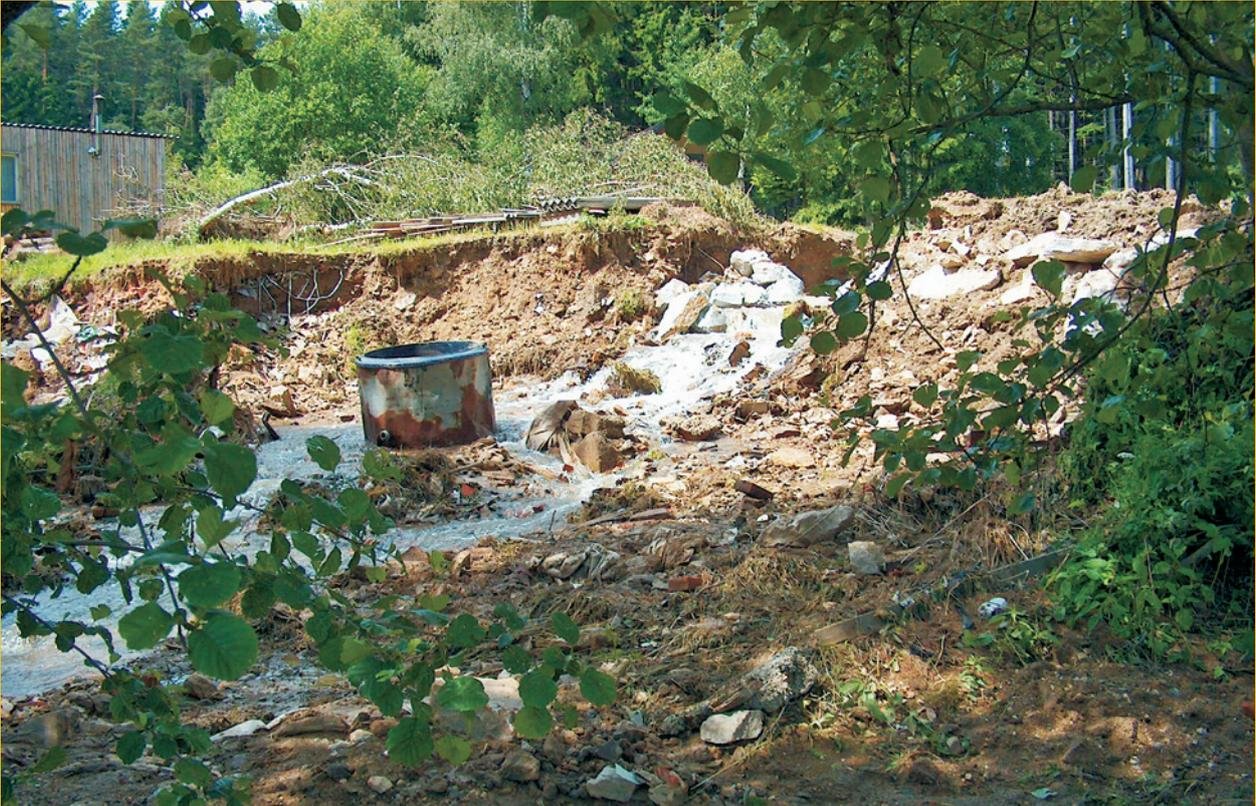
*Fig. 2: Partly destroyed dam of water reservoir after heavy rains in the upper part of the Olešenský potok brook watershed by Hlohov, Czech Republic (Photo: V. Vilímek)*
