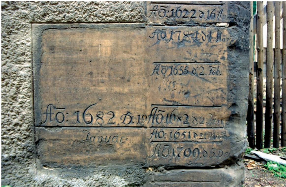
Fig. 13: High water mark of the extreme from 1 March 1784 in Halle (on the so called „New Mill“ in Mühlpforte Street) on the Saale R. as compared with other cases from the 17th century and from the beginning of the 18th century (Photo: M. Deutsch).
