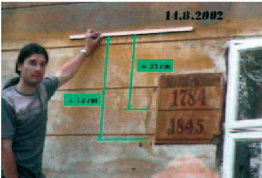
Fig. 7: Comparison of the Vltava (Moldau) R. water level in Prague reached on a Lesser Town house at the Charles' Bridge during the case in August 2002 with water marks of historical floods in 1784 and 1845 (Photo: J. Kubát).
