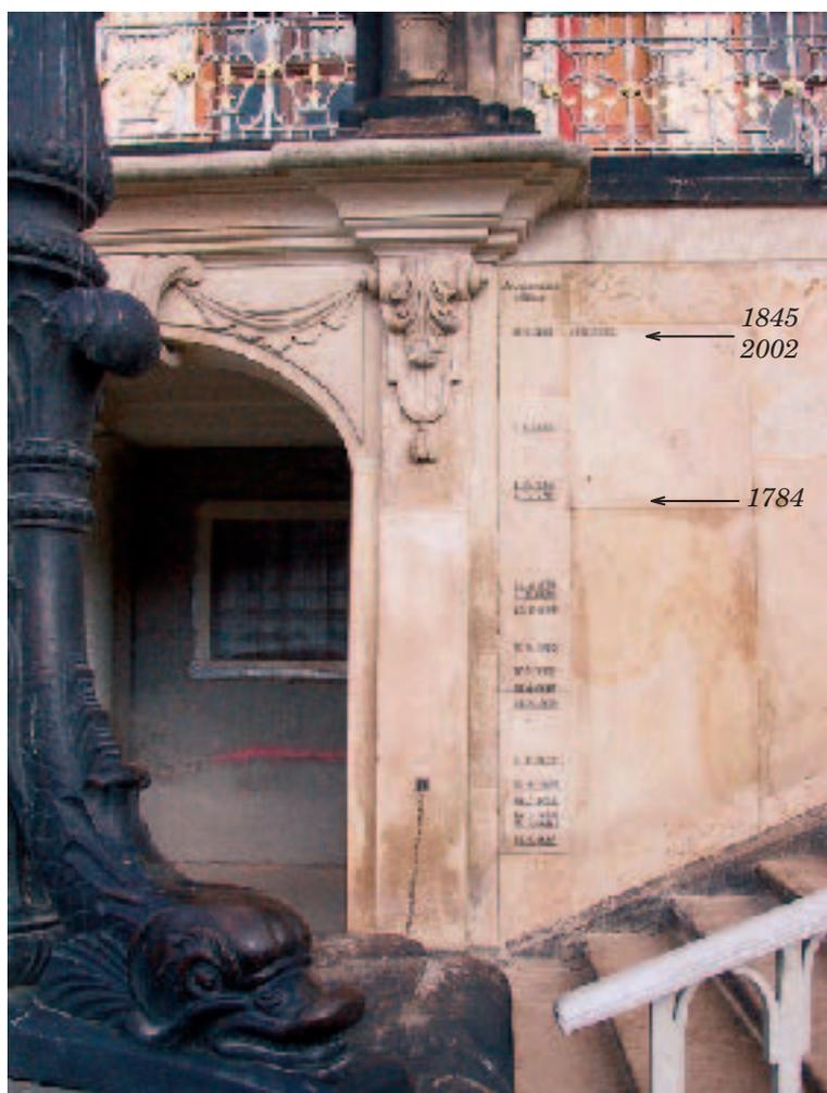
Fig. 11: High water mark of the extreme from 1 March 1784 on the water pavilion of Pillnitz Chateau near Dresden on the right Labe (Elbe) R. bank, and a comparison with the floods of 2002, 1845, 1890 and 1862 (Photo: U. Grünewald).
